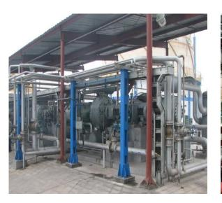
Coke oven gas compressor for steel mill
